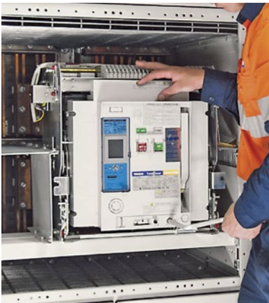
ACB upgraded with new Over Current Relay (top)
