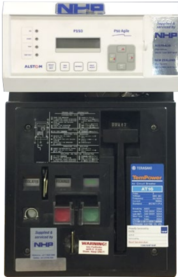
ACB upgraded with new Over Current Relay (top)
